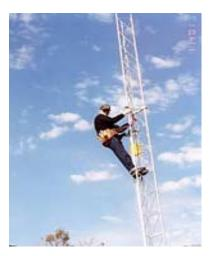
At present, the fourth section is up. I have finished the guy ends for the top. And the rotator is installed into the top section and checked out. Next step is to pull up the top section and guy it. Then the antenna can be set up. The regular
